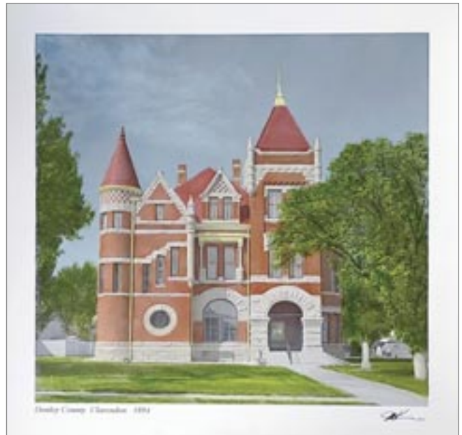
ABOVE: Handcolored photograph of the restored Donley County Courthouse in Clarendon taken October 2023. HANDCOLORED PHOTOGRAPH COURTESY OF JAMES MCKINNIS
