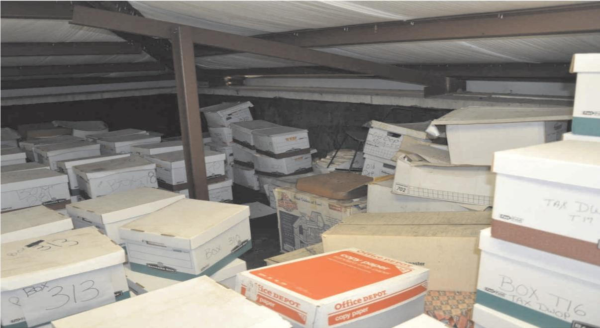
**PHOTO 73: Another Records room. Better view of the old roof serving as the floor and more collapsing boxes.**
